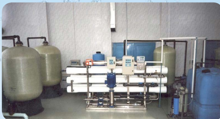
Water purification systems of Ecofil LLC used for treatment of extra-pure grade process water
